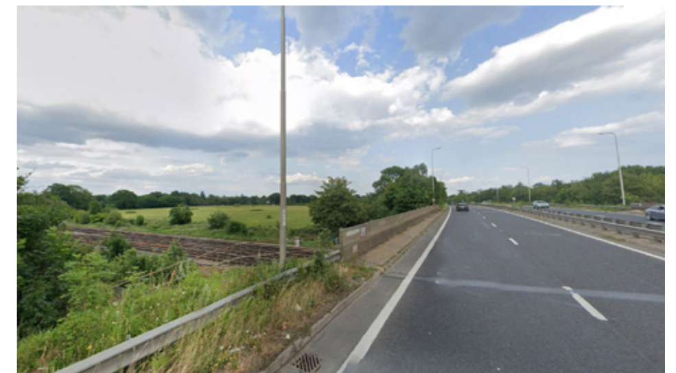
6. Airport Way looking towards site
